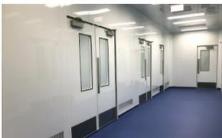
Spanning nearly 3,000 square feet, the GMP-compliant cleanroom includes 3 fully independent fill suites with their dedicated HVAC system and planned expansion for future needs. The layout includes personnel airlocks (PAL), material airlocks (MAL), pass throughs, eyewash stations, and dedicated areas for visual inspection, labeling, packaging, staging and cartoning. Flush-mounted windows and automatic opening doors complete the state-of-the-art installation.
